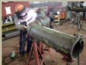
▼ Shuqaiq - Pipe Spool
