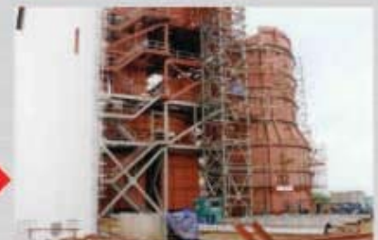
Krabi Power Project Installation of FGD System
